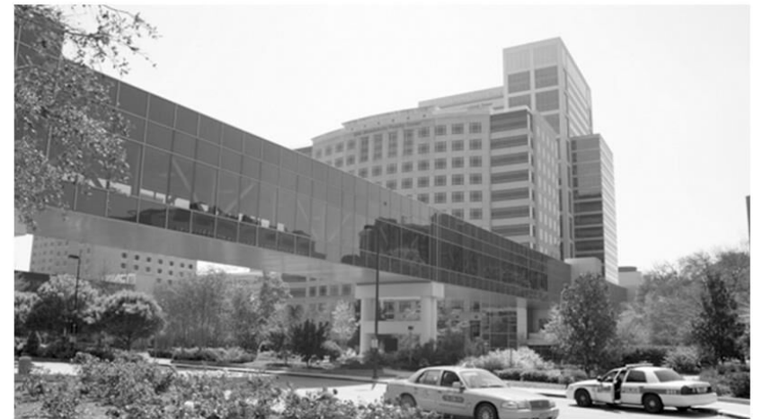
図 地上を介さず医療センター間を移動できる空中通路 (出典：Zheng Fang他「Case Study of Flood Mitigation and Hazard Management at the Texas Medical Center in the Wake of Tropical Storm Allison in 2001」)
